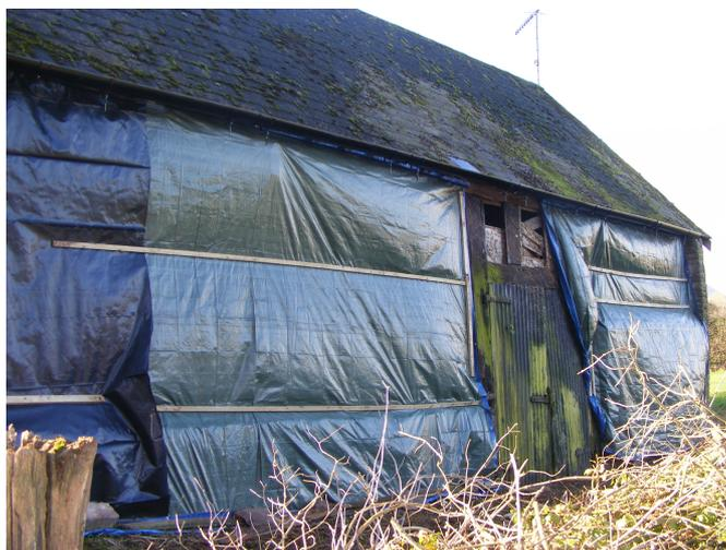
By late 2014, bad weather had further increased the vulnerability of the barn structure. Before knowing the outcome of the HLF bid, the Trust funded emergency measures to sheet the Barn to avoid further deterioration. Finally, with funds in place, the contractor, *Nigel Sobik & Son*, started the main contract work in March 2015.
