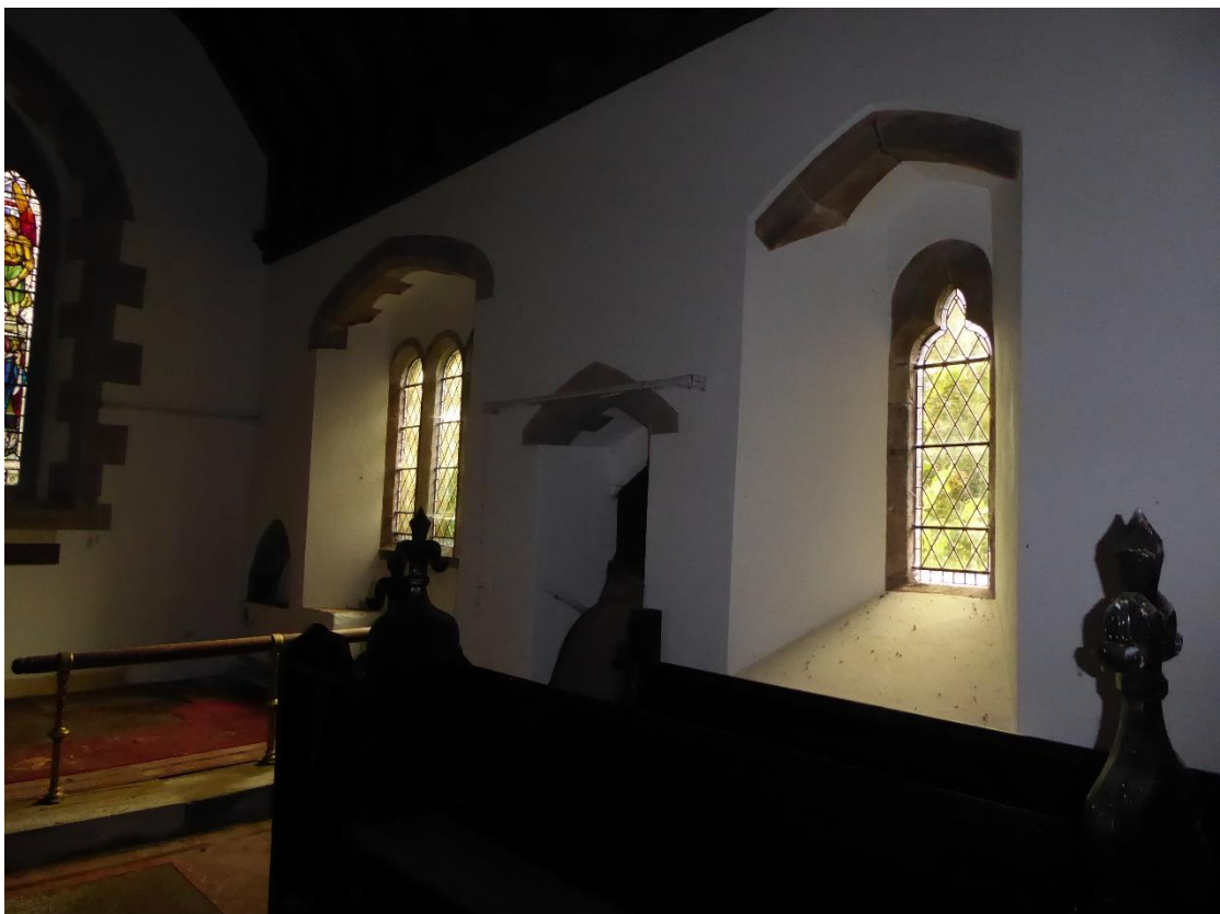
Fig 8 Chancel south wall
