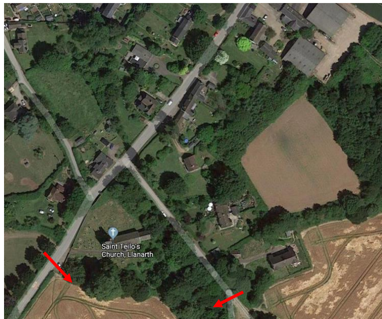
Fig 26 Aerial view marking potential for creating parking area © www.google.co.uk
