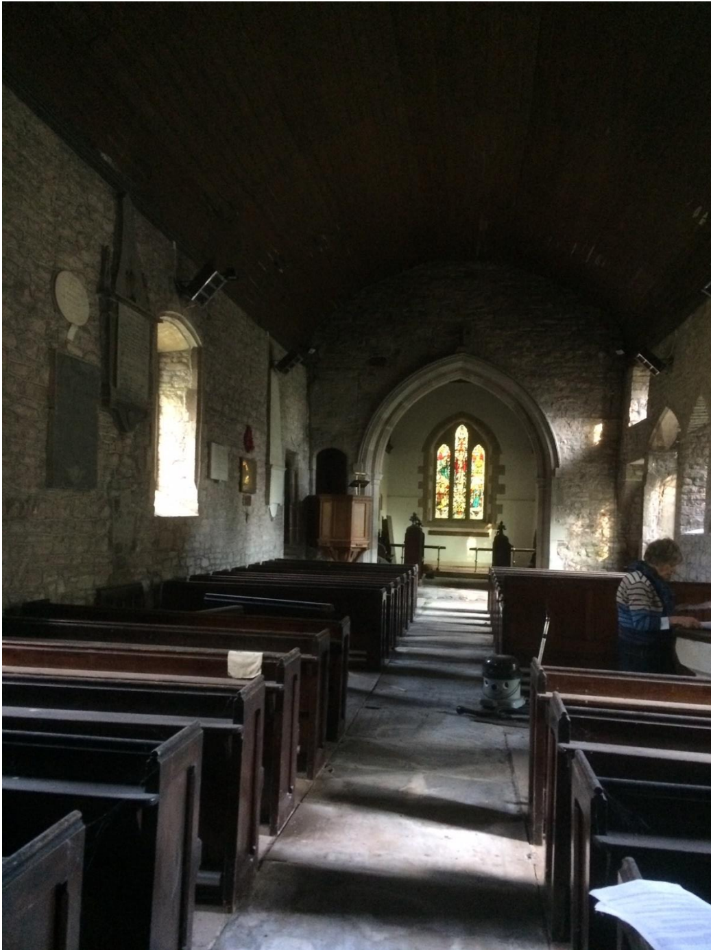
Fig 6 Interior looking east
