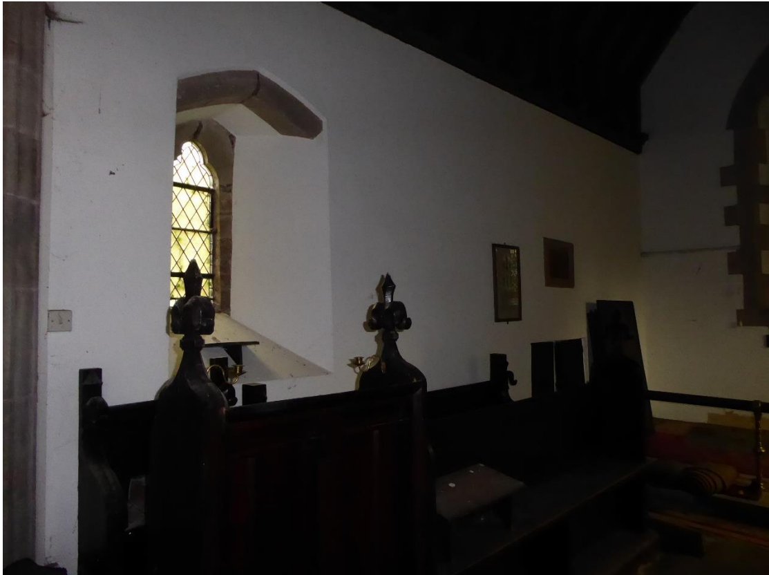
Fig 7 Chancel north wall
