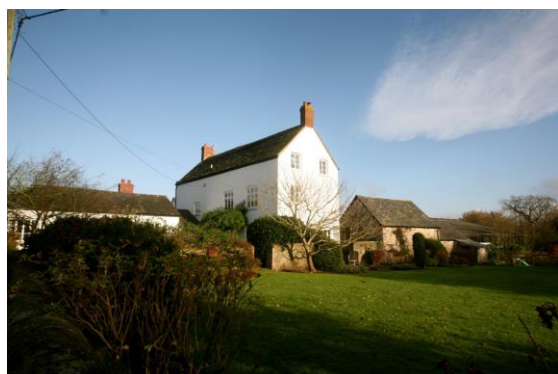
Fig.10 Church Farm comprises an important group of farm buildings to the edge of the village core
