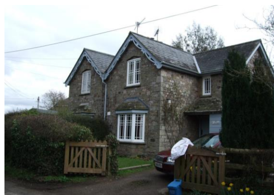
Fig.39 Nos 1-2 Pit Cottages distinguished by their large casements with margin lights and ornate barge-boards.
