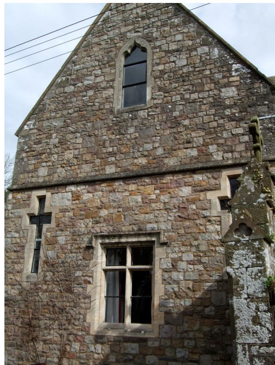
Fig.42 Mullion and transom or 'cross windows' distinguish Ysgol Clytha as the former Roman Catholic school
