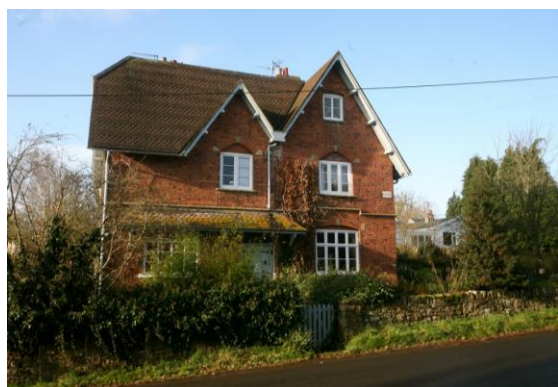
Fig.8 Bryn Teg. A pair of 'High Victorian' cottage scale houses in an early Vernacular Revival style at the core of the settlement
