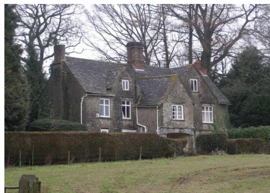
Fig.55 Pitt House. A fine example of a 17 th century gentry house, having gables, low profile, substantial porch, large chimney stacks and mullioned casement windows.
