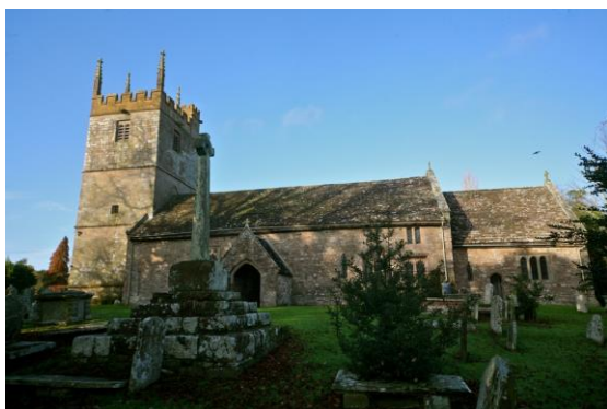
Fig.53 Church of St Teilo, from the south. The simple form of the church, without aisles or buttresses is apparent from this point of view at the junction with Heol y Ffynnon.
