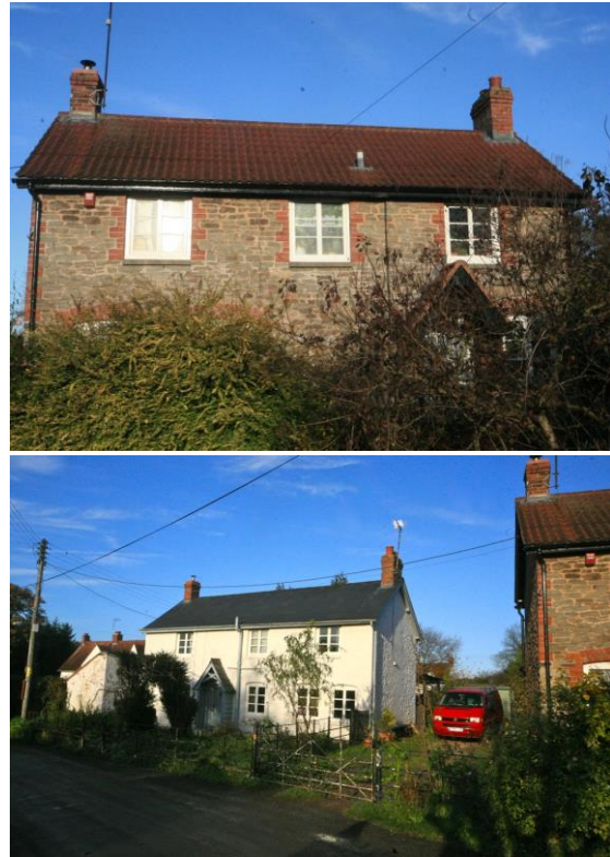
Fig.50 Nos. 5 & 6 are a distinctive pair, now differentiated by their roof coverings and wall finish
