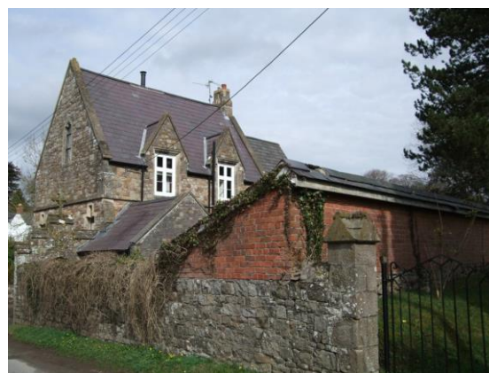
Fig.68 Natural slate in combination with rubblestone and red brick at Ysgol Clytha
